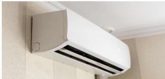
Gambar 2. 6 AC Split Wall
