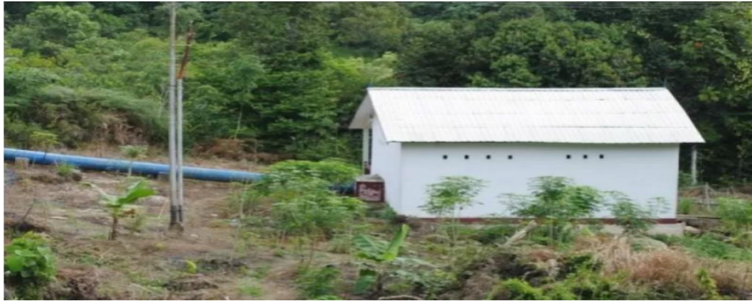
Gambar 2.8 Bangunan Power House
