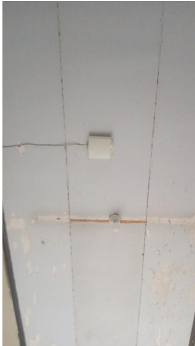
Gambar 3.25 Lab Mesin Access Point 2
