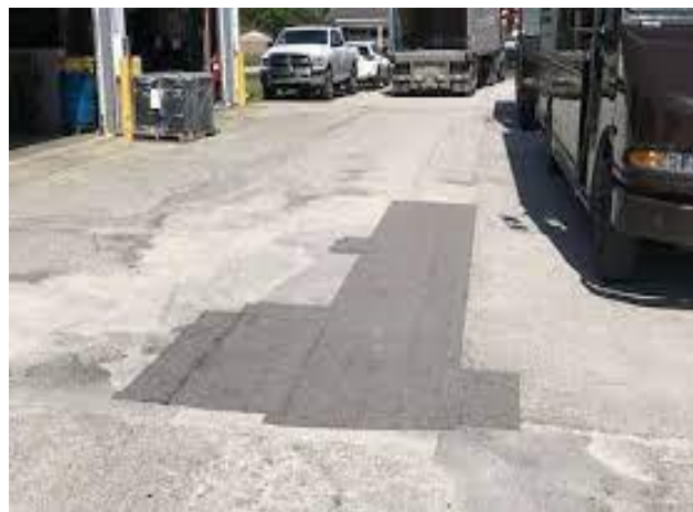
Gambar 2. 25 Tambalan ( Patching end Utiliti Cut Patching )
