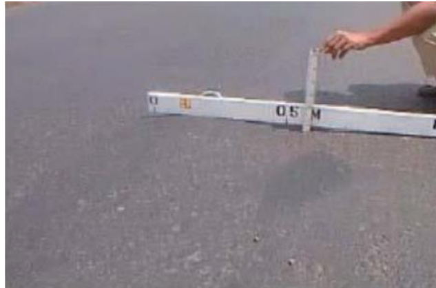
Gambar 2. 33 Alur ( Rutting )
