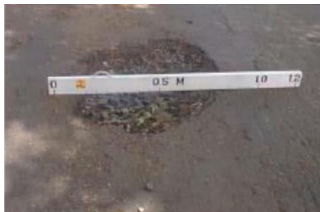
Gambar 2. 29 Lubang ( Pothole )
