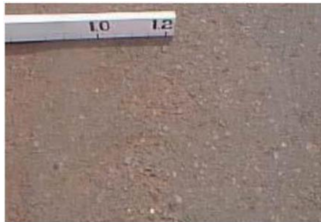
Gambar 2. 27 Pengausan Agregat ( Polised Agregat )
