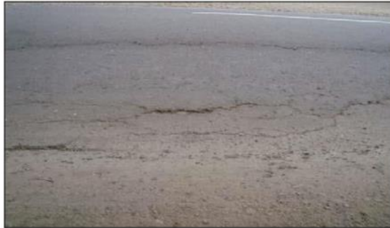
Gambar 2. 11 Cekungan ( Bumb and Sags )
