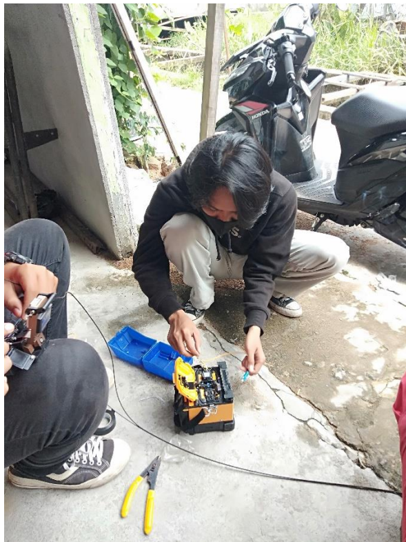
Gambar D.6 Join Ulang Patchcord Di User Jeruju
