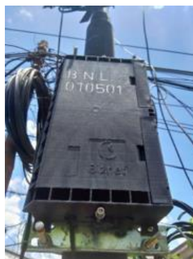
Gambar 2. 6 Optical Distribution Point Biznet
