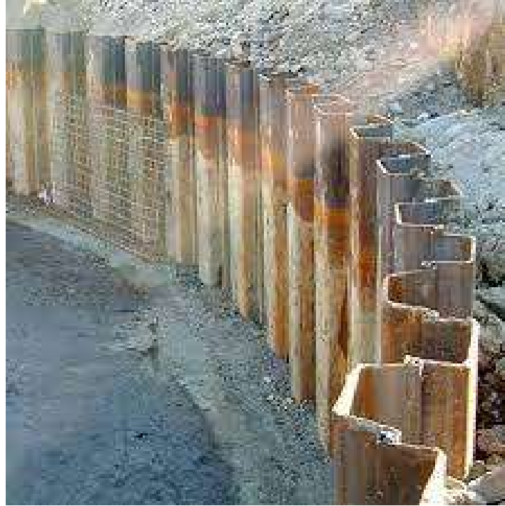
Gambar 2. 9 Steel Sheet Pile Wall ( www.designingbuildings.co.uk )
